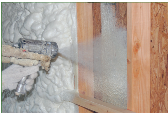
BioBased® Insulation being applied
