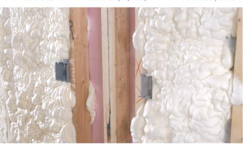
Airtight & Energy Efficient... Naturally Soy-Based Foam Insulation
